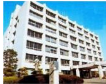
Board of Education (East Office Bldg.)
