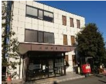
City Hall (Main Office Bldg.)
